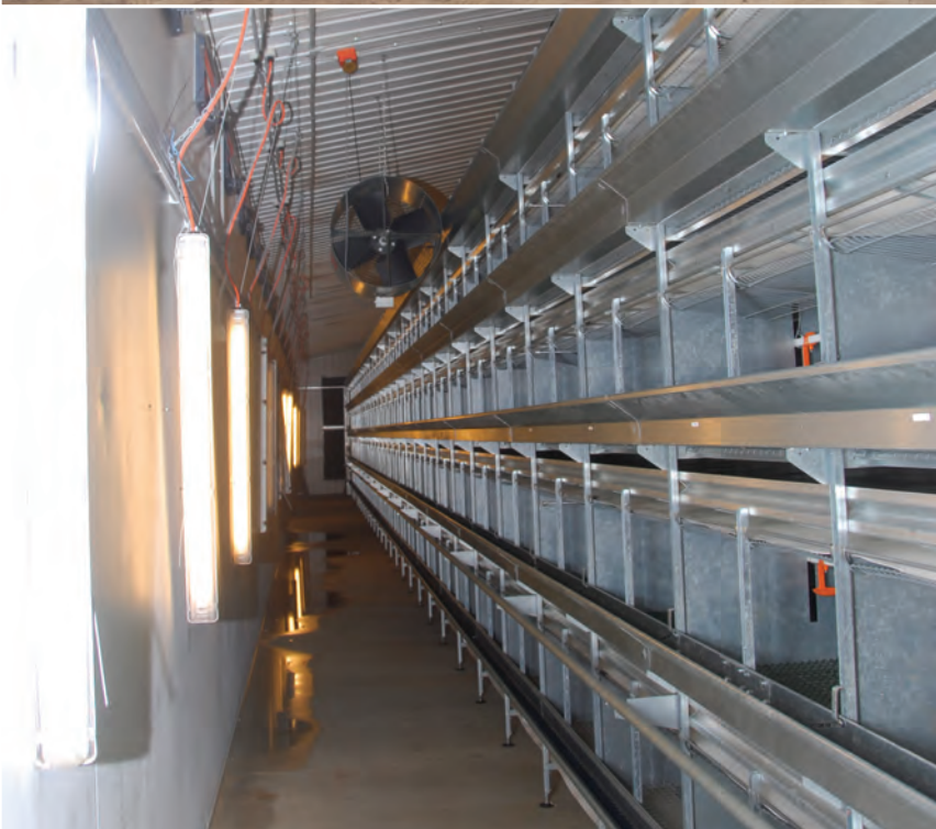
Top: Richard Dixon does a chick room temperature and humidity check. Particularly with layer pullets, chick room processing and holding temperatures are critical to ensure no overheating and/or chilling of the birds during the process. Centre: New shed R6 in expanded rearing unit. Above: Five tier Big Dutchman Eurovent starter cage system.
